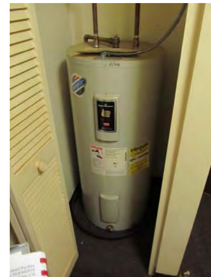
Electric, storage-type, tanks provide domestic hot water at each unit
