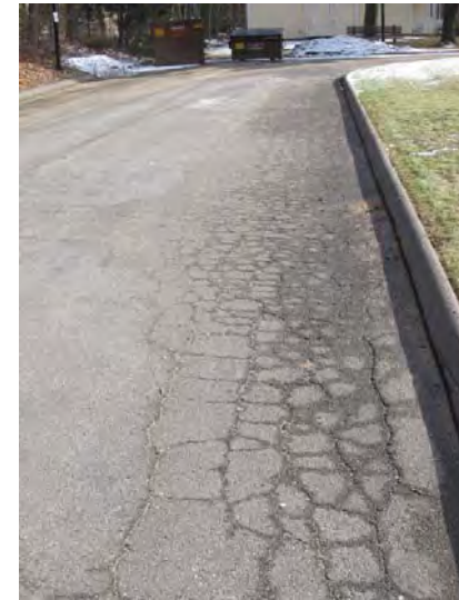
Asphalt paving on access drive exhibits cracks and deterioration
