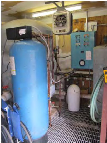
Components for well water system vary in age – No ongoing issues reported
