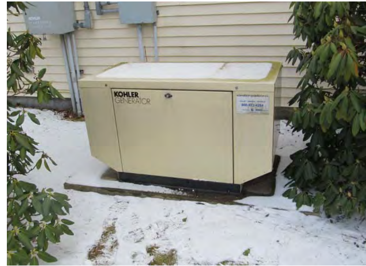
Propane-fired emergency generator at community building – Replacement not anticipated during timeframe of assessment
