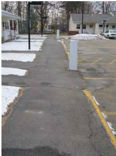
Cracks also evident at asphalt-paved pedestrian walkways
