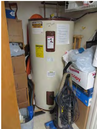
Electric, storage-type, domestic hot water tank serving interior common areas
