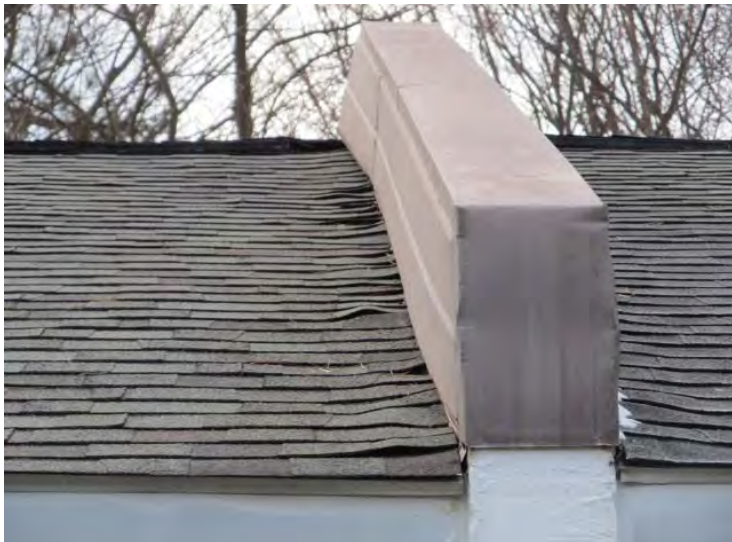
Roof shingles have been problematic and are not expected to achieve a standard service life
