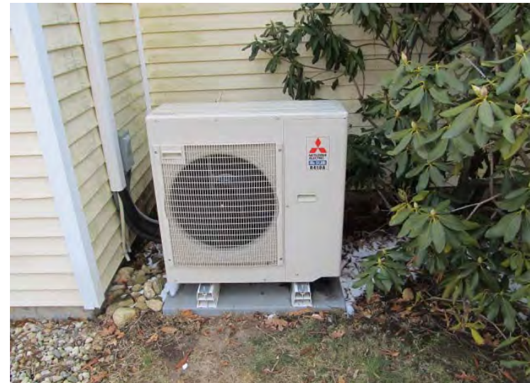
Exterior condenser for recently installed heat pump system at community building
