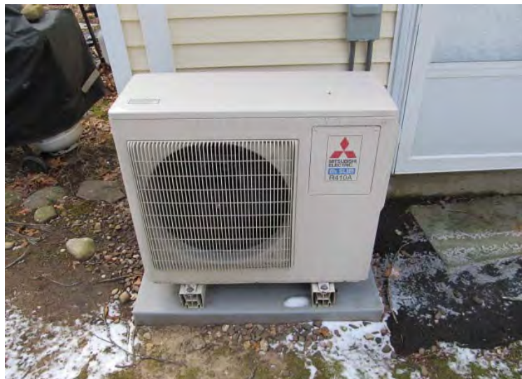
Typical, exterior-mounted, condenser at each unit that serves the recently installed heat pump system
